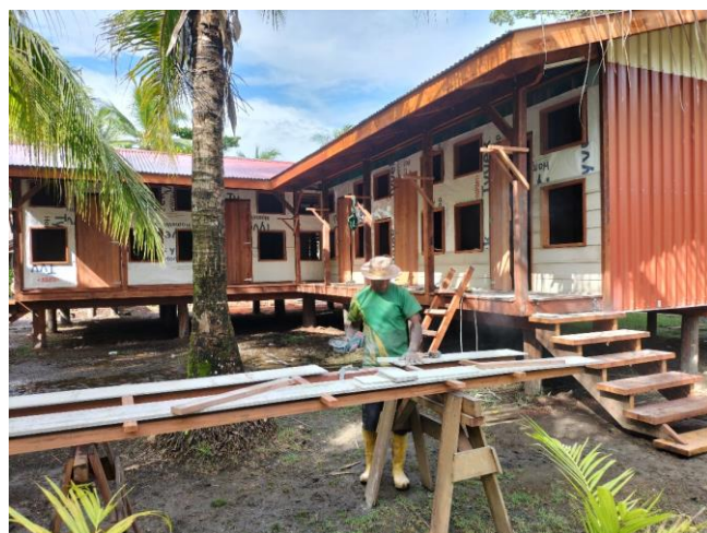
The dorm under construction. Doors are in place, windows are framed and cladding is being cut.
